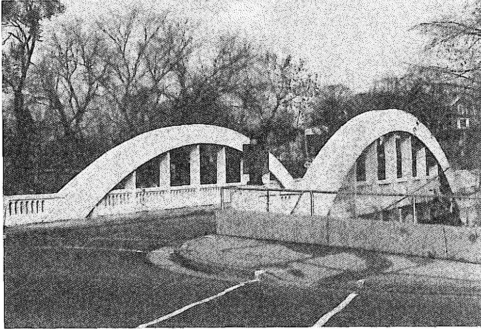
FIGURE 6 Reinforced concrete rainbow (or Marsh) arch bridge (1916). (Wisconsin DOT photo.)
