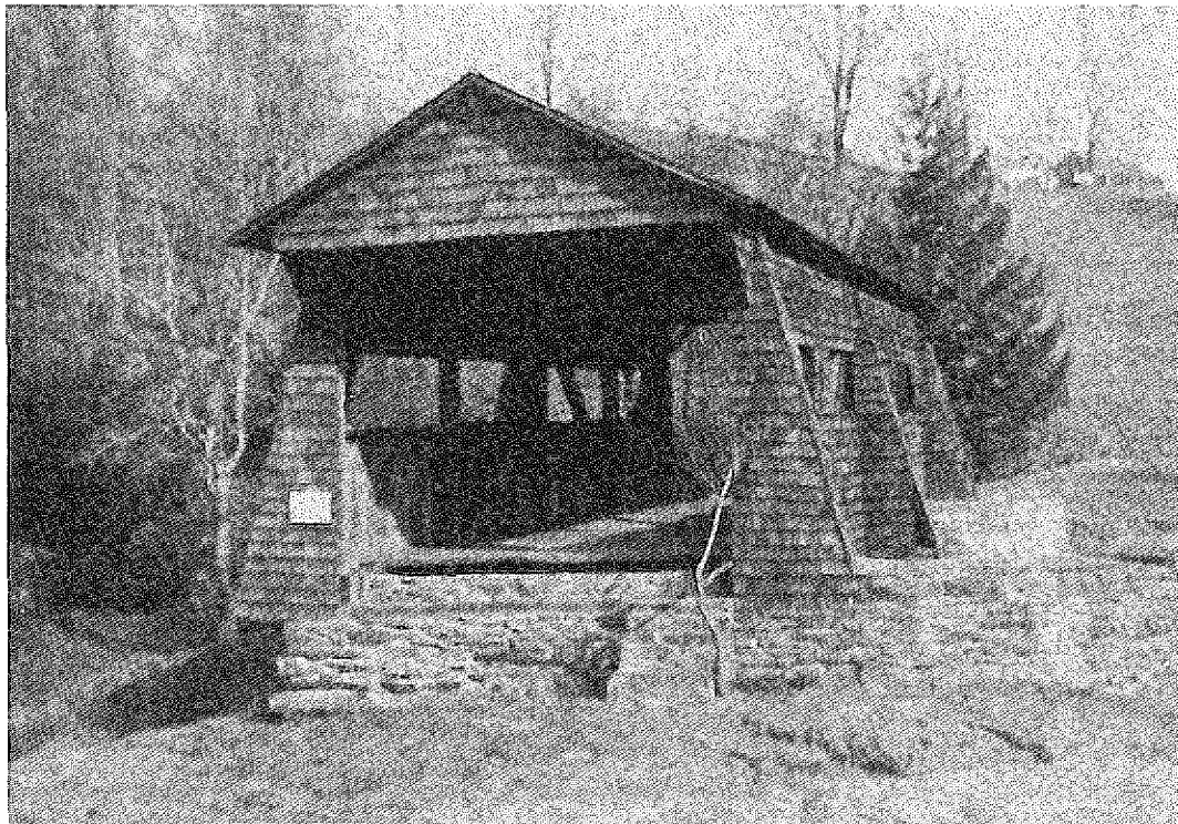
FIGURE 11 Tuscarora Club Bridge (1870), Delaware County, New York, was moved in 1935 from Donraven, New York, and re-erected on a private preserve for fishing access. (Richard S. Allen photo.)
