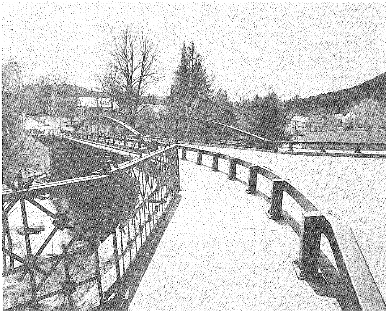
FIGURE 7 Elm Street Bridge (1870), Woodstock, Vermont, showing the restored Parker trusses incorporated into the replacement structure. (Clay Gates photo.)
